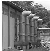
An exhaust and ventilation system is used to reduce exposure to airborne pollutants by drawing out air containing pollutants within an indoor area and replacing it with fresh air from the outdoor. The centrifugal fan controls the flow of air in the indoor area by drawing air in from the outdoor, and pushes airborne pollutants or stale air out from the indoor area.
