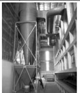
A cyclone dust collector system is used to enhance the quality of air by removing dust particles and other airborne particles from industrial processes.
