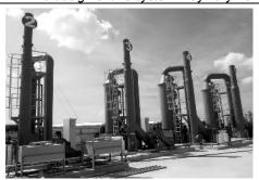
A scrubber system is used to remove gaseous pollutants such as chlorine fumes, sulphur fumes, nitrogen fumes, cyanides, ammonia and odour produced as by-products from industrial processes. Among the major types of scrubbers that we manufacture are counter-current scrubber, crossflow scrubber, venturi scrubber and chlorine emergency scrubber.
